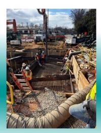
**CULVERT FINAL CONCRETE POUR COMPLETE**
