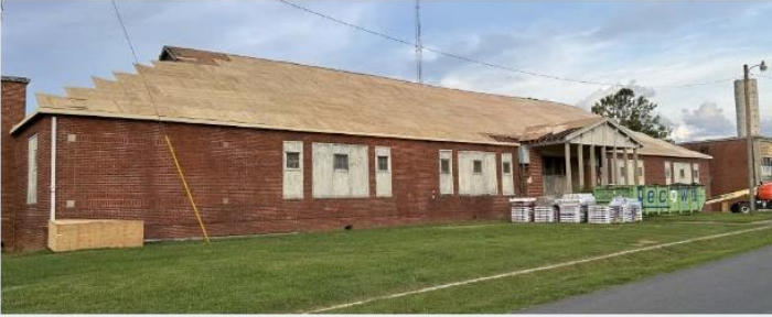
Torrence-Lytle High School Roofing Project
