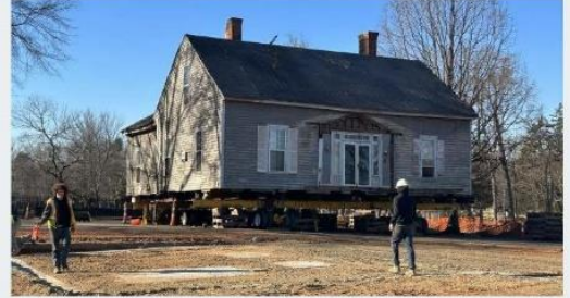
Relocation of Douglas House
