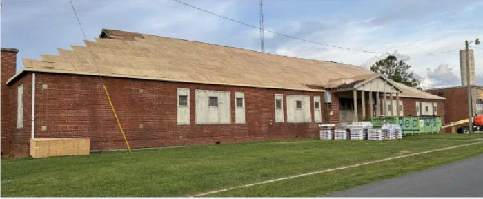
Torrence-Lytle High School Roofing Project
