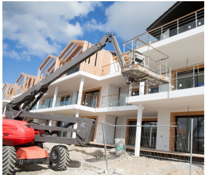
Townhome Construction, Public Domain
